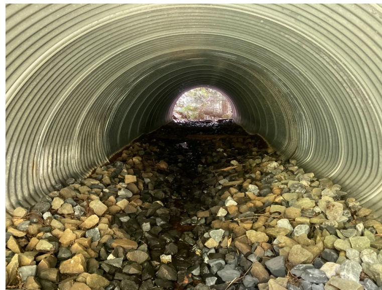
Looking Downstream Through CMP
